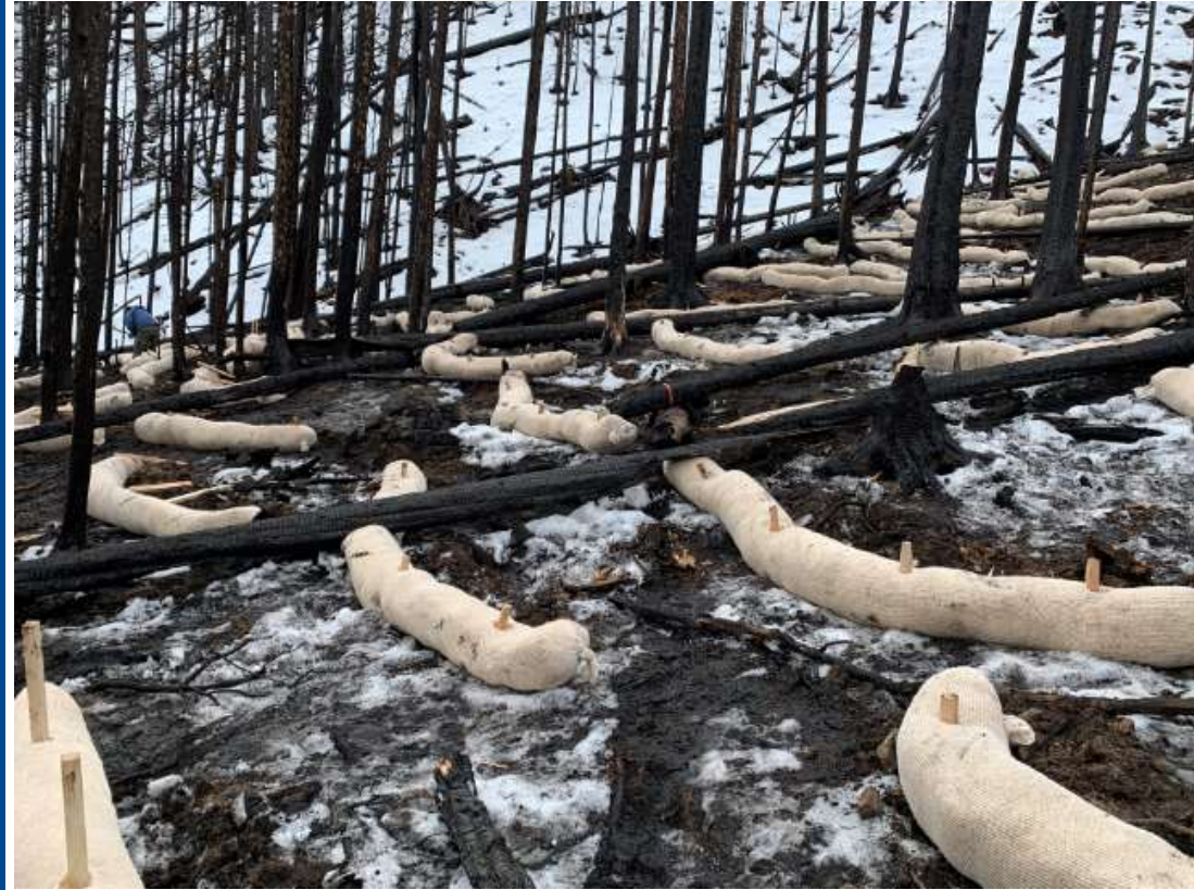
Wattles installed at Chambers Lake for slope stabilization
